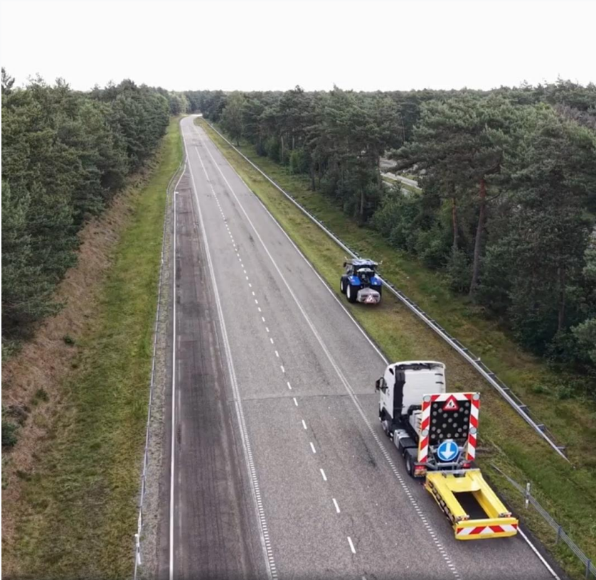
Mobile worksite scenario on the Lommel motorway track
